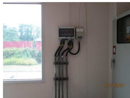
Chlorine Gas Leak Detector
